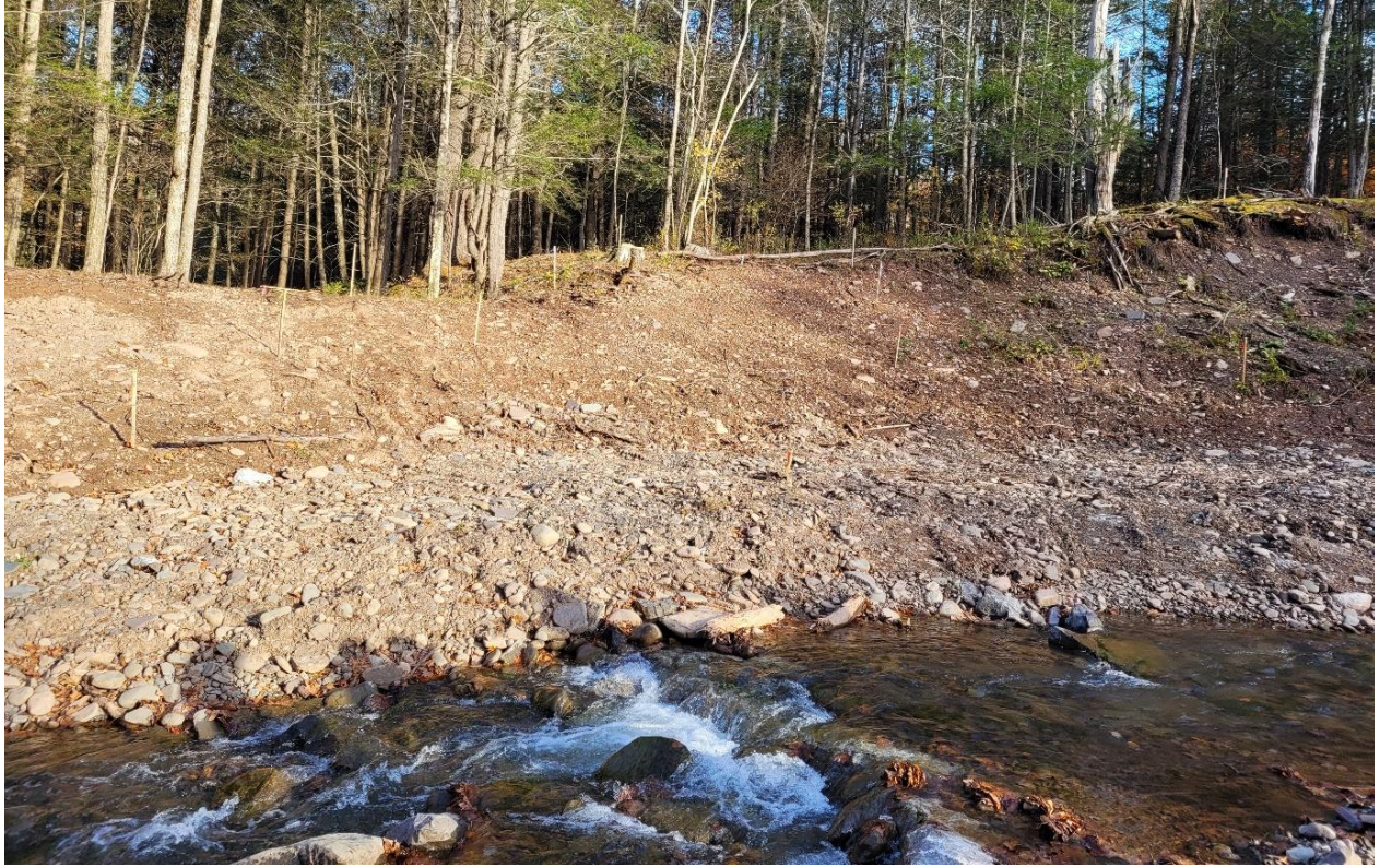
Figure 1. Panther Kill Stream Restoration Site in Woodland Valley. The Panther Kill sediment turbidity reduction project (STRP) is one of a dozen in the Catskills that have been constructed since 2012. The STRP at Panther Kill was near completion in the fall of 2022. Photo taken by C. Swanson on October 28 th , 2022.
