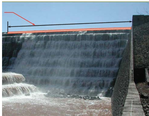
Figure 14. Placement of the notch (arrows) that was removed from the Gilboa Dam (NYC DEP 9, 2007).
