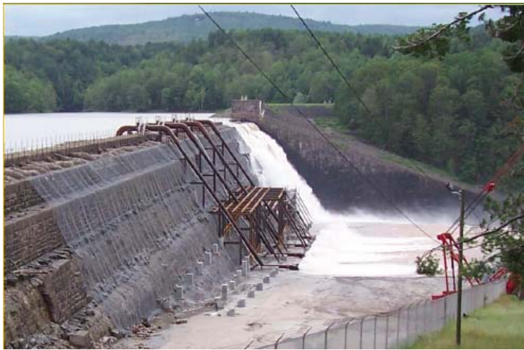
Figure 15. Gilboa Dam after the siphons were installed as part of the NYC DEP's short term reconstruction (NYC DEP 9, 2007).
