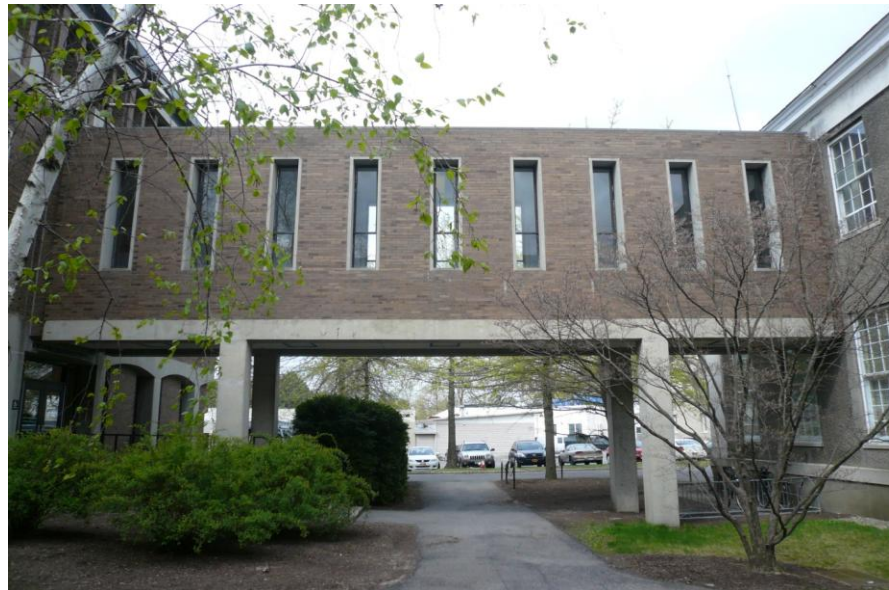
Figure 9: “Bridge” connecting Science and Engineering North to Steinmetz. Note the trees and vegetation around windows, as well as the fact that one can see from one window through the parallel window.
