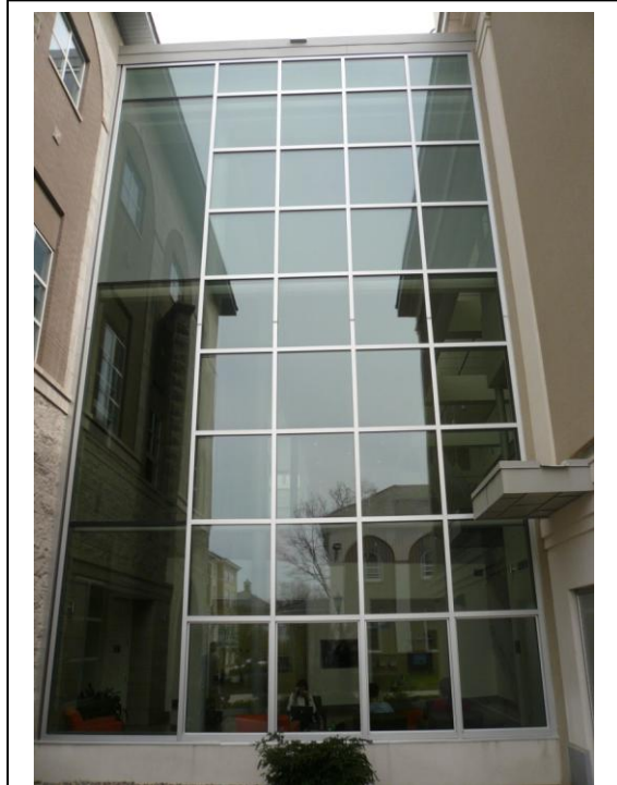
Figure 8: West facing windows in Peter Irving Wold Center. Note that only the top portion of the window is fritted.
