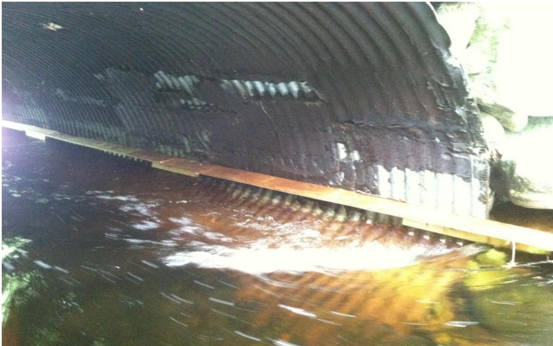
Figure 2. Ledge (5½” wide) with support blocks installed in Sucker Brook culvert, Edinburgh, NY. Also represents atypical flash flood June 2013.
