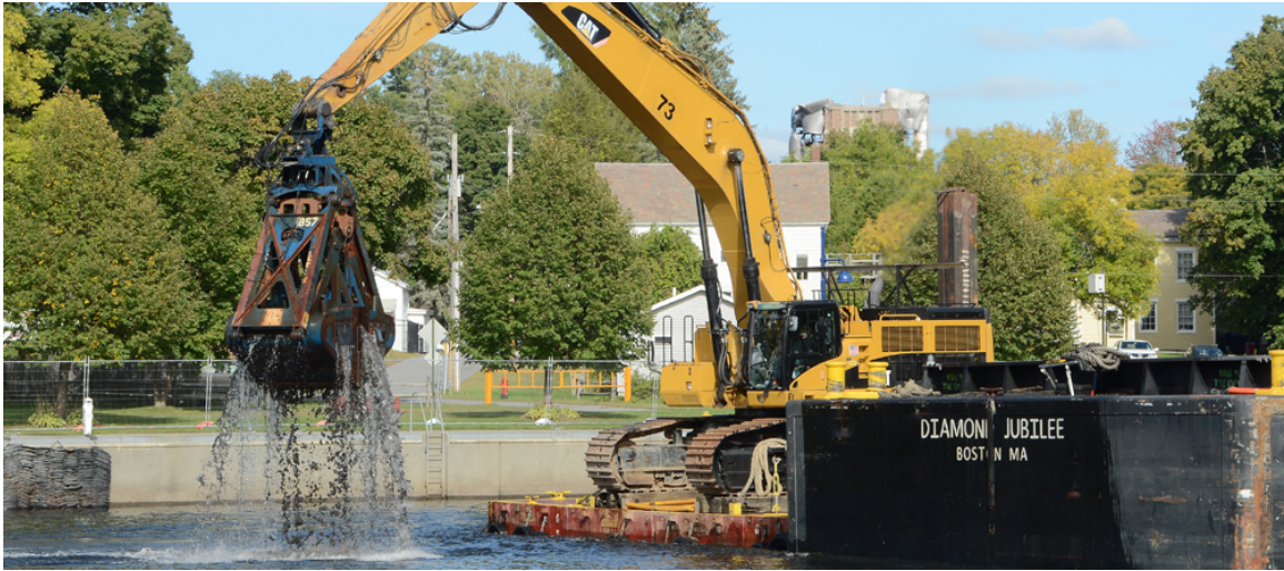
Figure 8. Equipment used by GE during Phase 1 dredging (The Hudson River Dredging Project. “A Historic Achievement”, 3/7/16).
