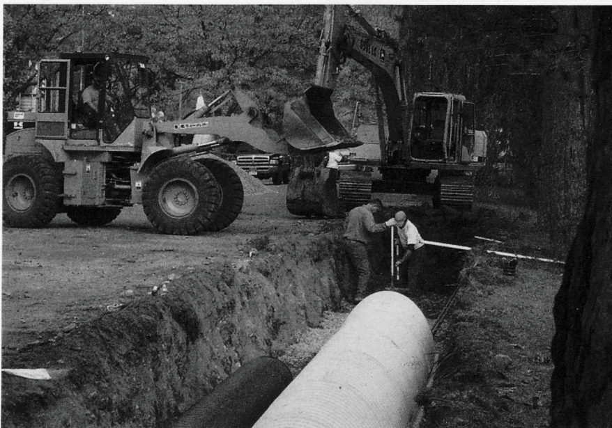
Installing a stormwater runoff infiltration chamber system to protect Lake George from polluted runoff.
